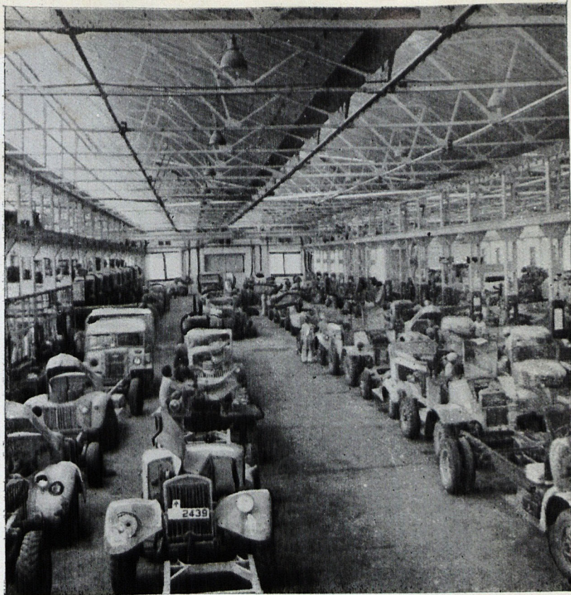
Army lorries under repair and overhaul in an I.E.M.E. 4th Line Workshop.
